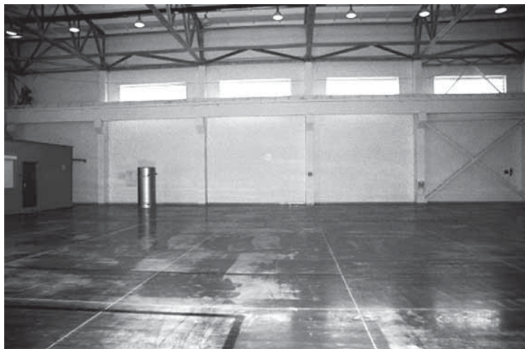
Fig. 1.4. International Uranium Enrichment Center’s storage facility at Angarsk Electrolysis Chemical Combine.
