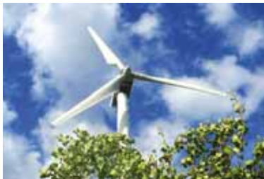
Windmill installation in Murmansk ▲ (photo: Bellona)
