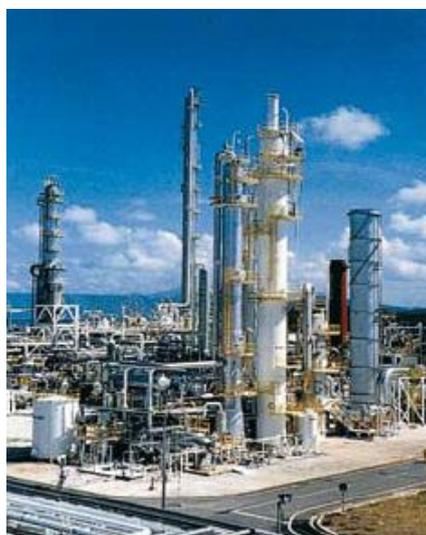
**FIGURE 1. INSTALLATION FOR POST-COMBUSTION CAPTURE OF CO<sub>2</sub> FROM FLUE GAS. SOURCE: IPCC.**
