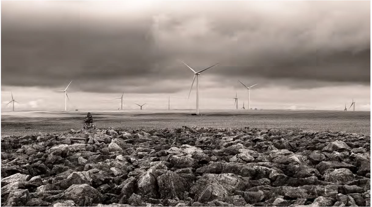
Varanger Kraft's Raggovidda Wind Farm in Berlevåg, Finnmark (Photo: Varanger Kraft)
