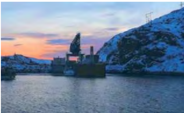
Kislogubskaya tidal power plant (Foto: OAO «Malaya (Minor) Mezenskaya Tidal Power Plant»)
