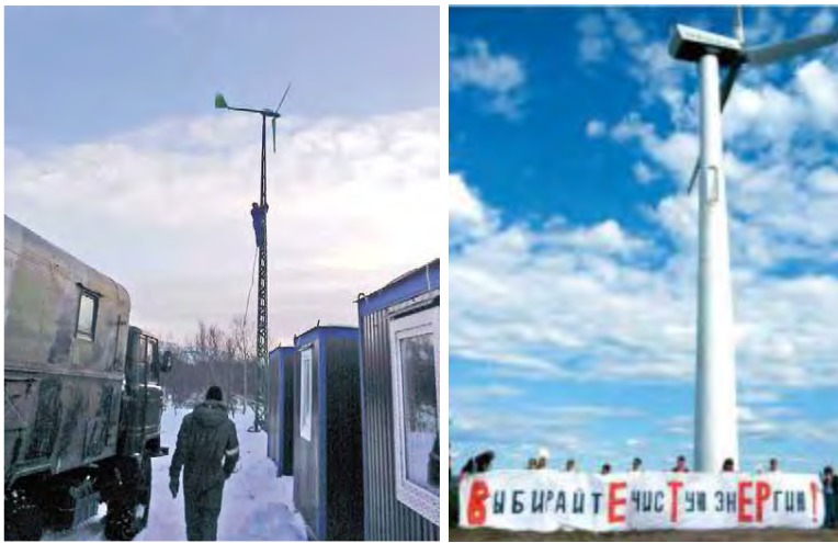
Left: Wind power installation in Novaya Titovka, 9 kW (Foto: ООО «Murmansk») Right: Choose Clean Energy! Wind power installation in Murmansk (Foto: Bellona)
